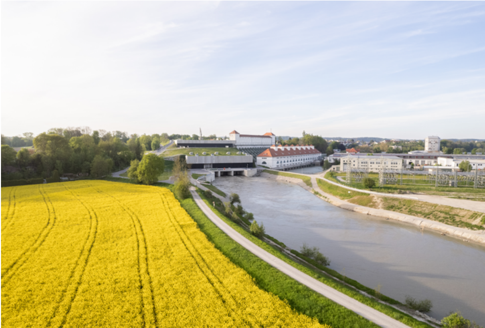
Töging hydropower plant: The new plant (centre) has been in operation since 2022. The old plant can be seen on the right (summer 2023).
