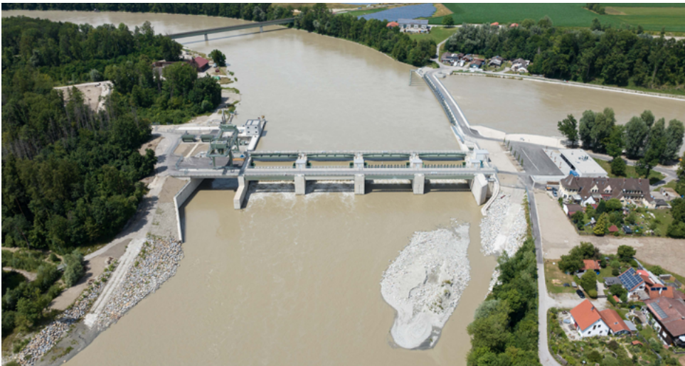
Jettenbach weir: The newly built weir on the Inn River controls the inflow of water to the run-of-river hydropower plant.
